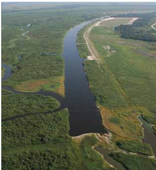
C-38 canal, pre-construction, source from:
