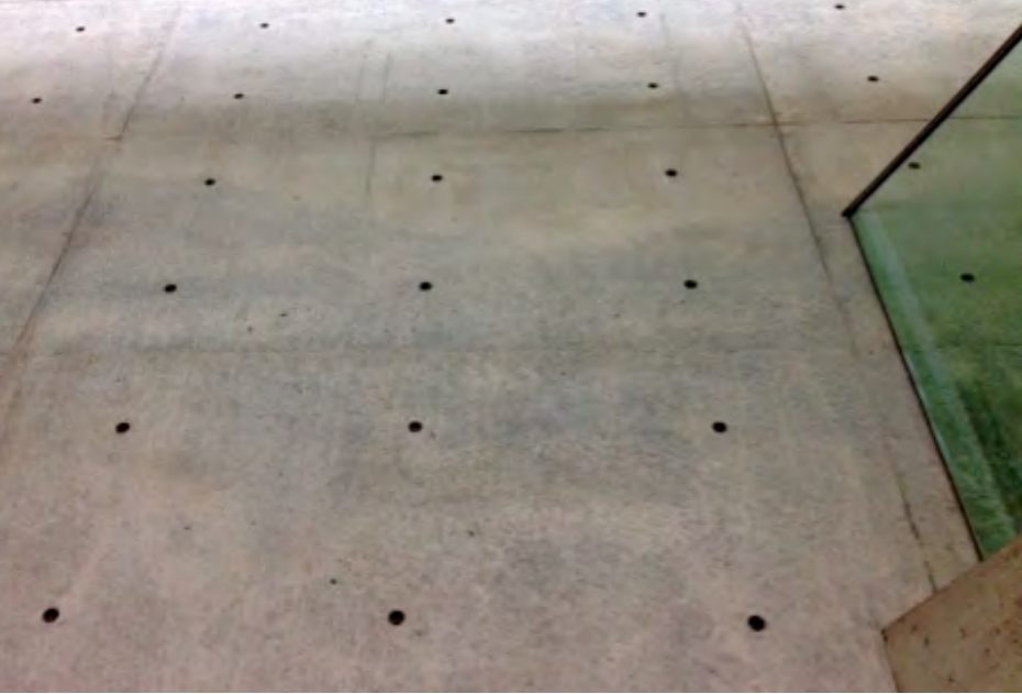
Figure 6. Use of the Osaka Standard fair-faced concrete in the AMMA, each slab is the same size of Japanese Tatami.
