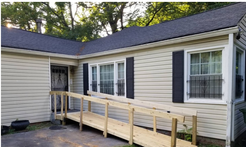
This was a wheelchair access ramp for a disabled senior. We replaced a heavily damaged ramp with this new one, along with fixes to her driveway to ensure she could enter and exit her home.
